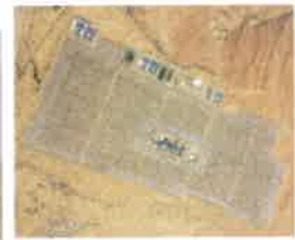
"Ashalim" (Israel) 120 MW, 338 lazos 1500MWth (~4.5h)
