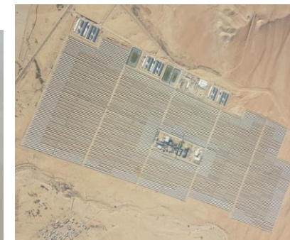
“Ashalim” (Israel) 120 MW, 338 lazos 1500MWth (~4.5h)
